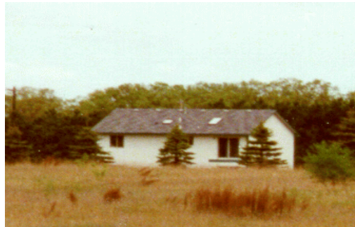
Fire hazards of this home include tall grass
