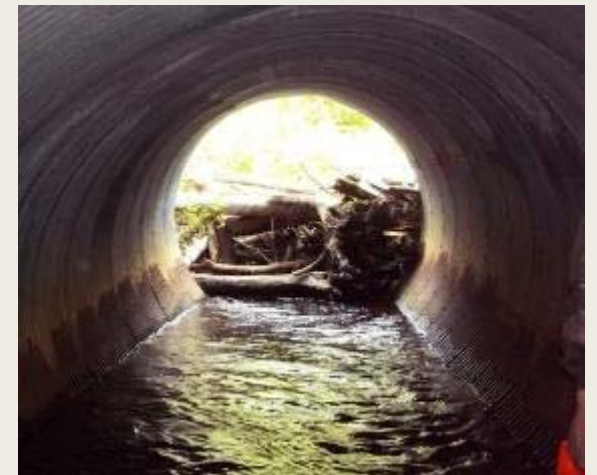
Blocked Culvert
