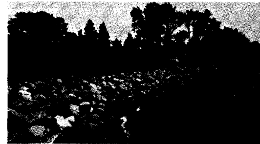
A rubble-mound revetment was installed on Madeline Island in Ashland County to help protect an Indian Cemetery of historical significance. The revetment was used here at this low-bluff and narrow-beach site.
